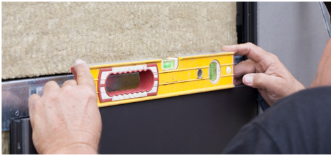
5 The installer ensures that the panel is level.
