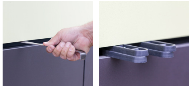
8 Minor adjustments can be made to the panel spacing. Spacers can be used to ensure consistent spacing between panels before they are attached to the framing system.
