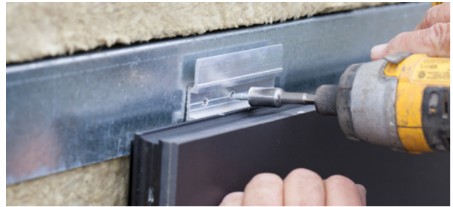
6 The aluminum clip is attached to the sub-framing using a self-drilling hex screw with an extended hex head driver.
